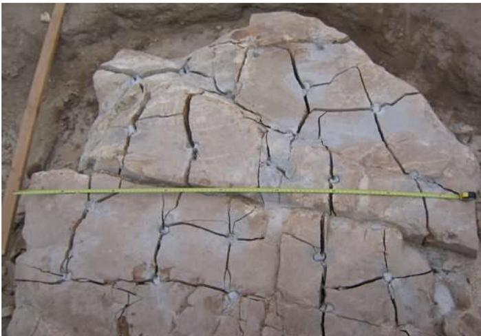
*Figure 1: Rock cracked by using expanding cement, Dexpan (2015).*
