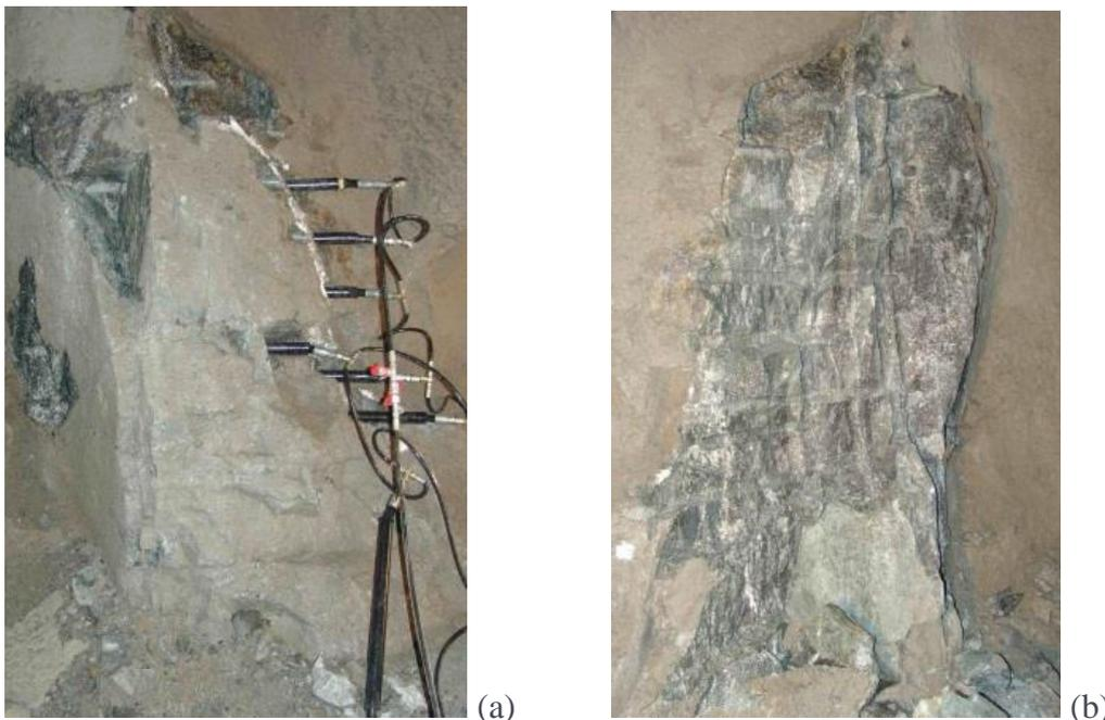
*Figure 33: (a) Arrangement of the splitters; (b) after removal of the under-break*
