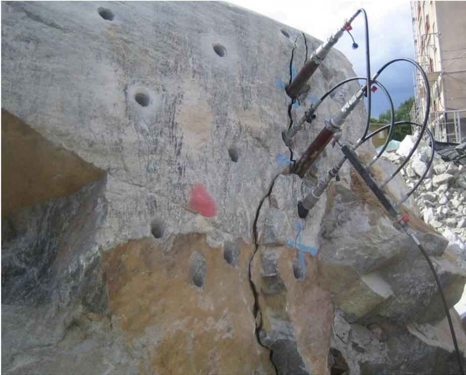
*Figure 36: Splitting a large rock block at construction site New Karolinska Hospital*
