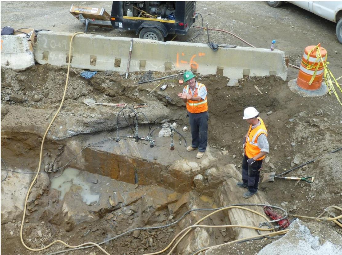
*Figure 35: Splitting a vertical rock wall with a free surface, Manhattan, New York*
