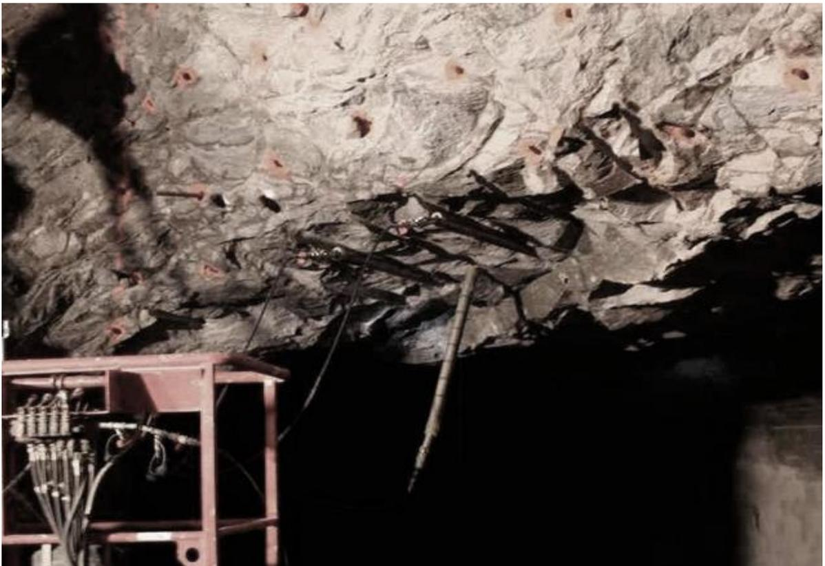
*Figure 34: Splitting the tunnel roof in City Link project in Stockholm*
